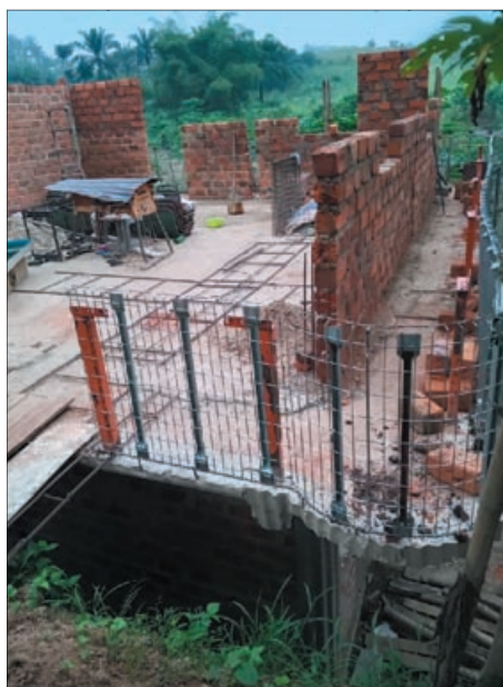
Protective railing all around the second floor ...Raising the walls
