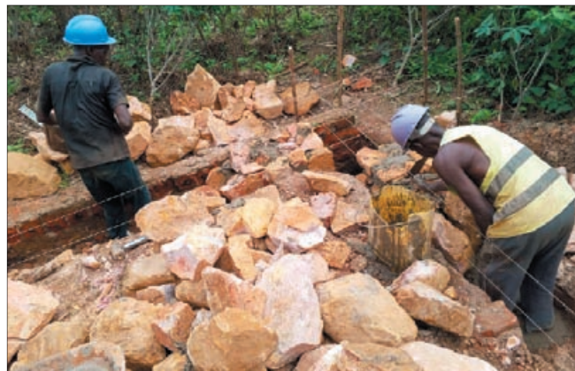
Digging, measuring, preparing pillars, mixing stones and cement
