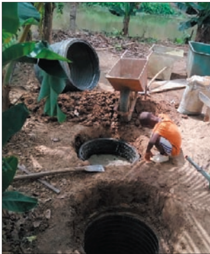
Construction for fish breeding
