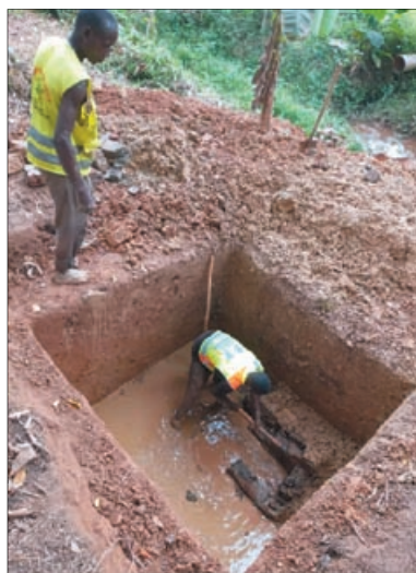
Digging 7 meters deep for the well
