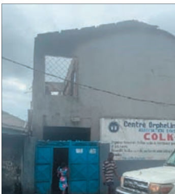
The top floor of the COLK orphanage burned down completely because of a faulty electric system
