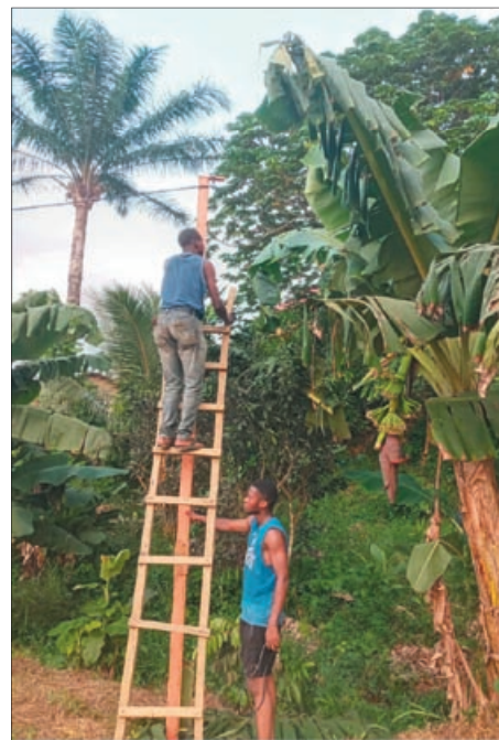
Attaching the cable to 6,5 meter high poles, deep in the farm ...
