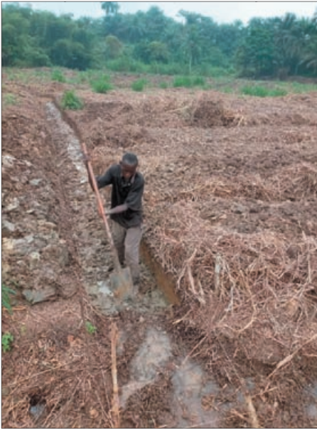
Digging ditches against floods
