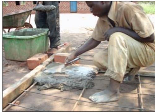
*Water reservoir constructed (l), cement ceiling formed (r) and finished (below)*
